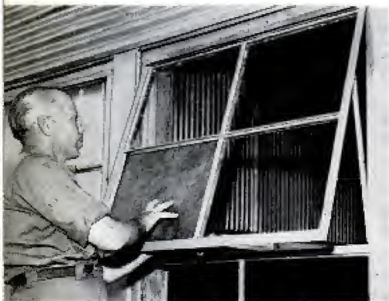
Absolutte Company of America photo Above, flat-type translucent plastic may be used in place of regular frosted glass where vision is not desired. Below, panels of corrugated plastic, 10 or 12 ft. long, simplify construction of a carport roof
